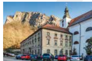
Pohled od severozápadu View from the north-west
